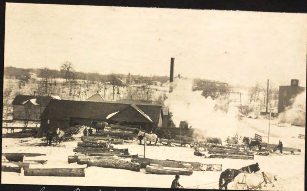
Saw Mill, Hanover, Minn. 1906
