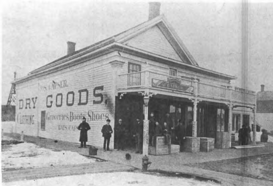
Figure 2: Moore-Capsler Building, 1879 (Sinclair Lewis Interpretive Center)
